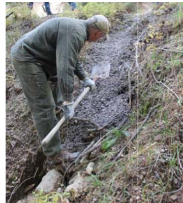
Figure 4. Upstream gully being manually armored with Zerosion to stop roadbed undercutting and side-slope washout.
