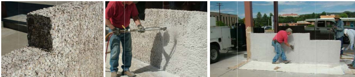
Figure 6. The different steps in building with Chipcrete.
