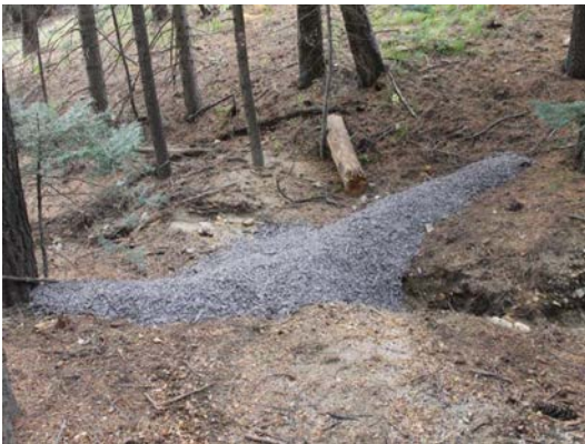
Figure 3. Downstream berm to slow and spread water coming down steep embankment for AZ Department of Transportation trial.
